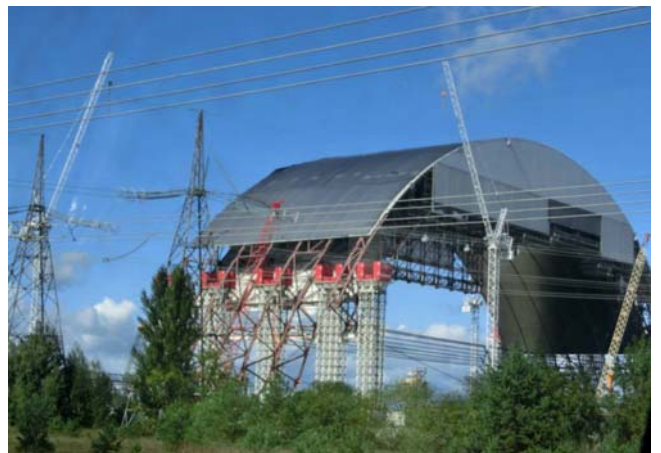
Fig.5 Chernobyl-Unit 4, New Safe Confinement ("ARCH")
